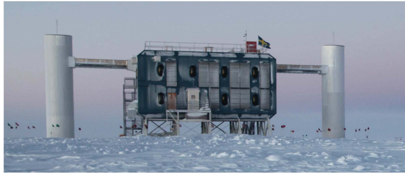
Figure 1. The IceCube Laboratory building houses power, communications and data acquisition systems for IceCube and other experiments at the South Pole (photo by Sven Lidström, IceCube/NSF).
